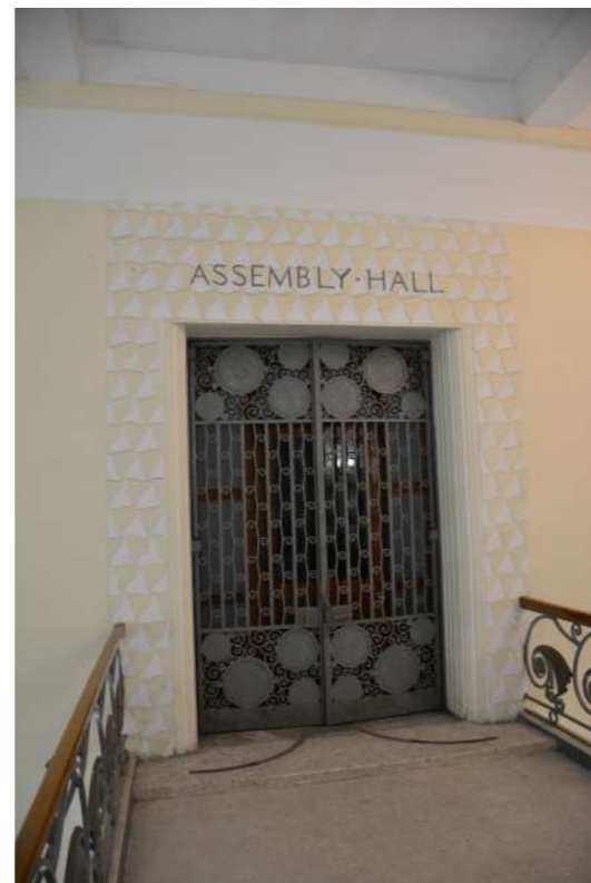
Fine detailing to the entrance of the Arts Building Assembly Hall
