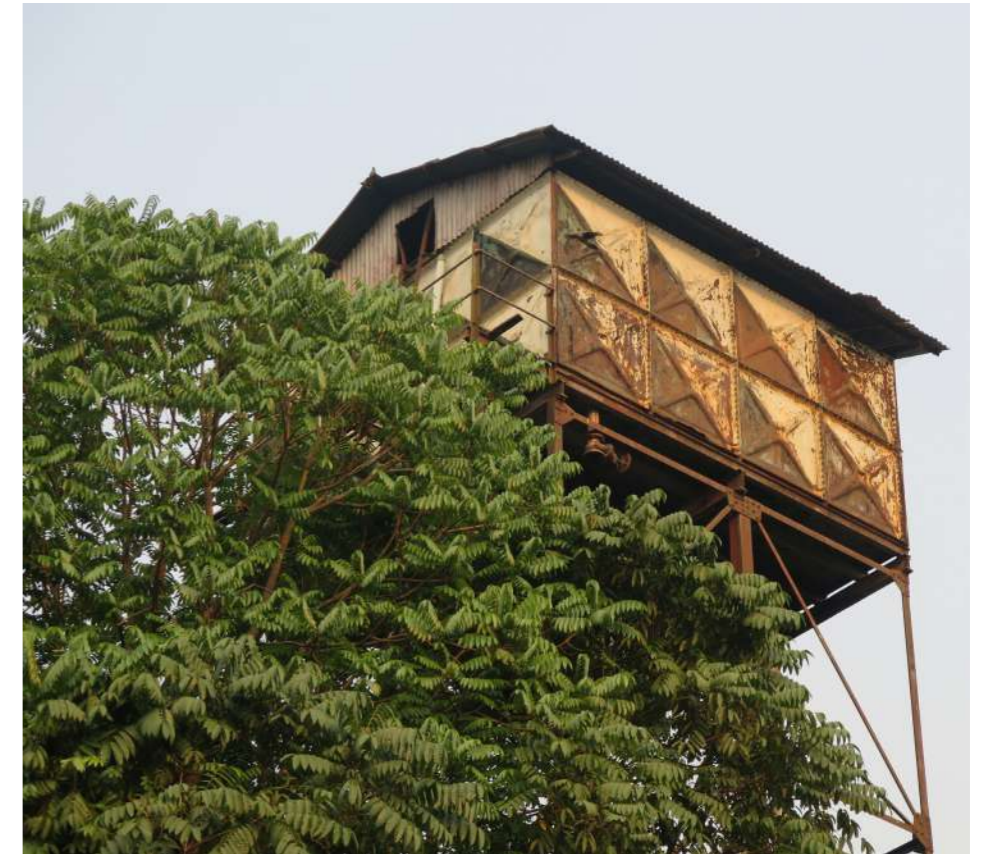
Steel water tower, Kamayut Campus
